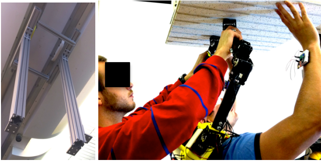
Figure 6. Figure to the left shows the test rig where the ceiling panel has to be installed. Figure to the right shows one of the trials where test subject #2 (wearing red) helps test subject #1 during the ceiling panel installation task. As shown in the figure to the right, two IMUs are located at the test subject #1's wrists.
